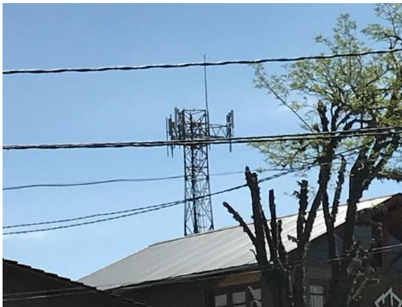
Communications Tower (3 km away)
